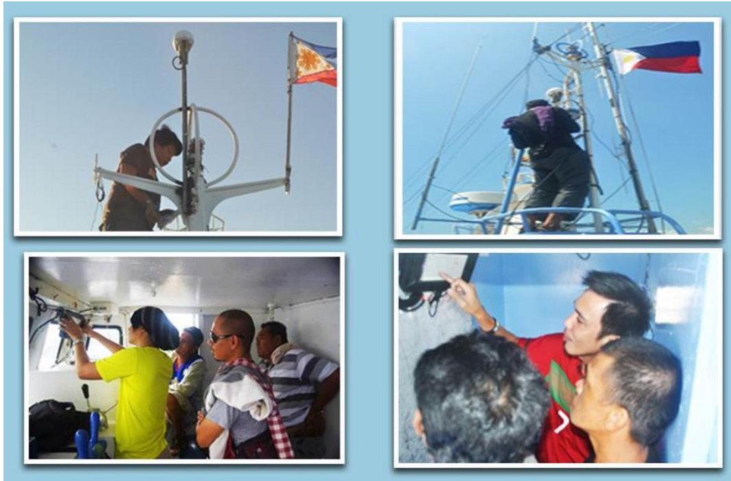
Fig. 1. Installation and trial operation of MARLIN onboard catcher vessel including VMS MTU.
