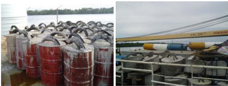
Figure 12. FAD anchors constructed of concrete filled steel drums and concrete anchors loaded on a ranger vessel ready for deployment
