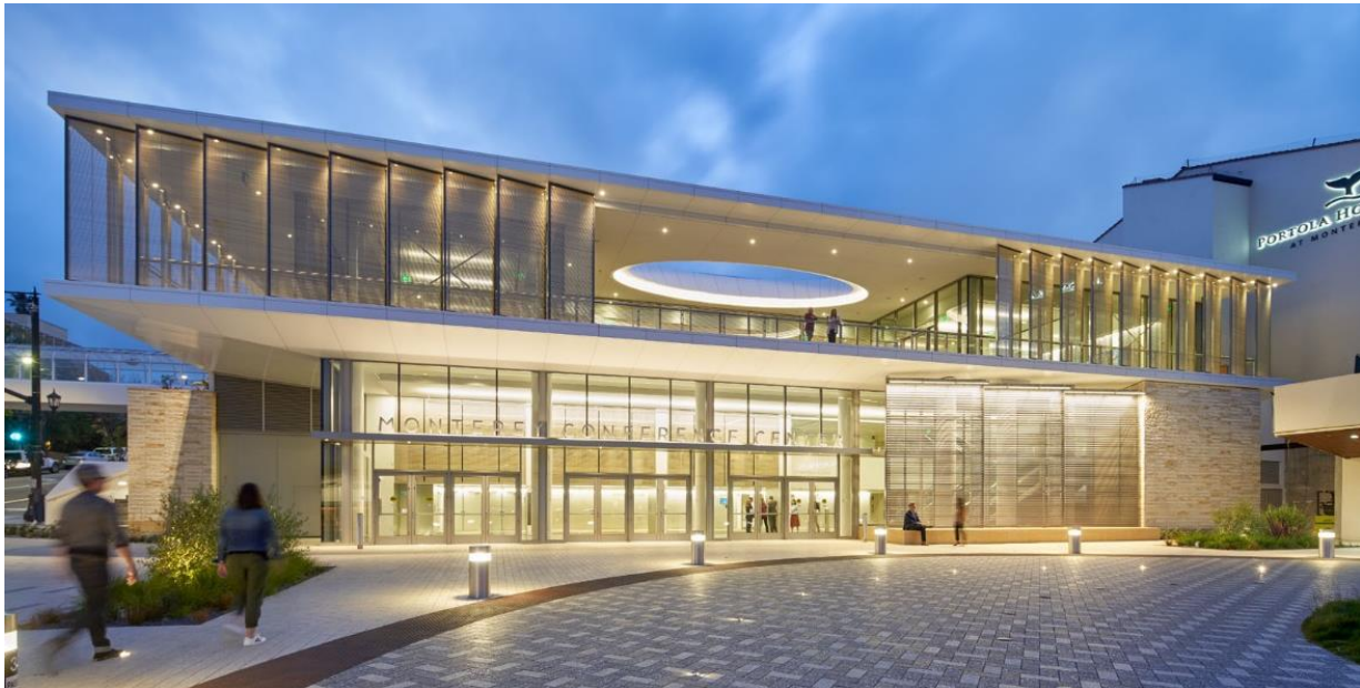
Monterey Conference Center and Portola Hotel & Spa at Monterey Bay
